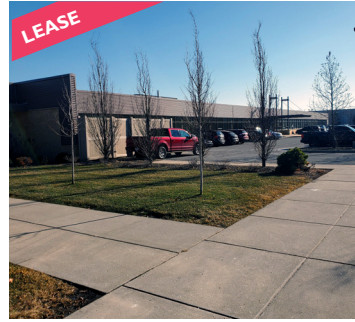
LAKE BUSINESS CENTER OFFICES 9200 CALUMET AVE, MUNSTER, IN
