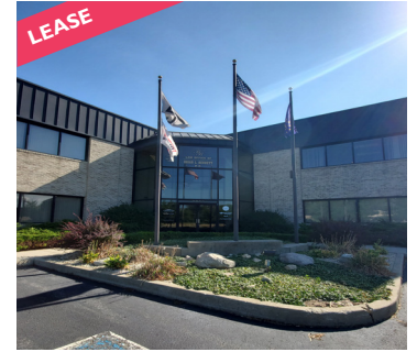
LEASE OFFICE 2803 BOILERMAKER CT. | VALPARAISO, IN
