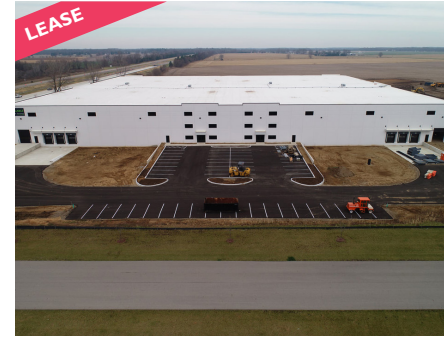
SBDV IV - UNDER CONSTRUCTION NORTH DYLAN DRIVE, SOUTH BEND IN 46628
